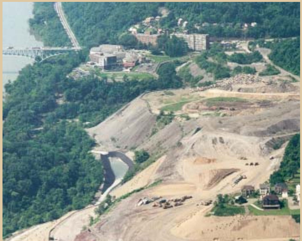
In Pittsburgh, before brownfields cleanup, this slag pile occupied a spot near Frick Park above the Monongahela River.
