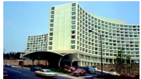
Concrete has long been a part of hotel construction, as shown here at the Capital Hilton Hotel in Washington, D.C. completed in 1942. Photo: Portland Cement Association
